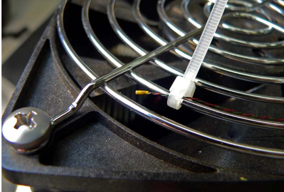
Small sensor on the finger guard of a fan in an area of high air flow
