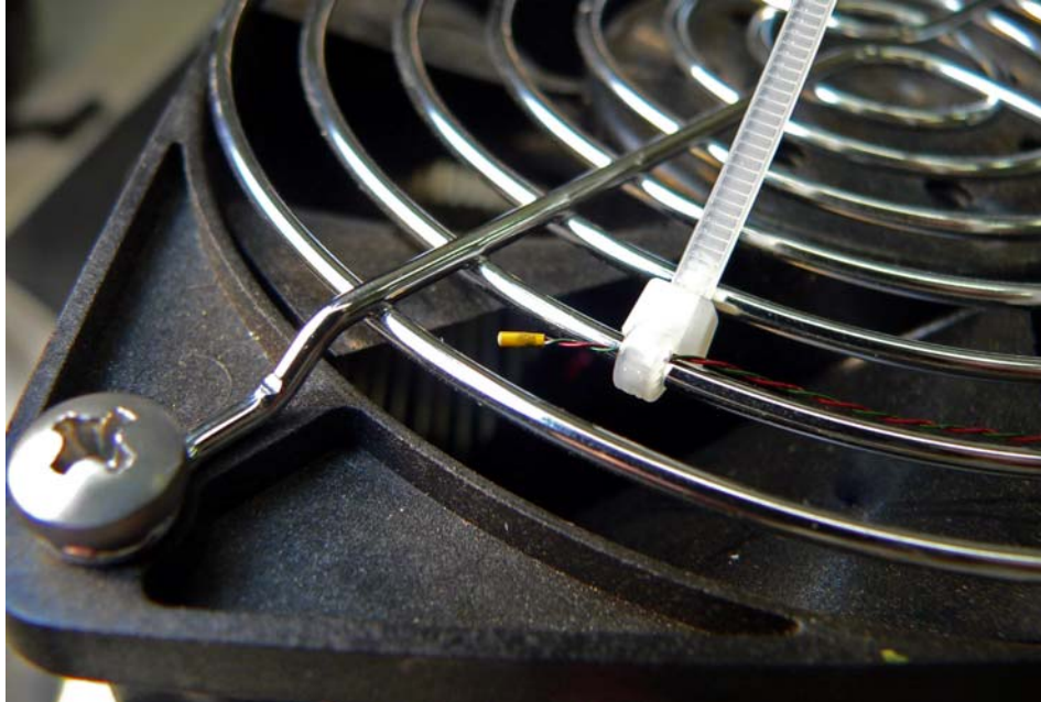
Small sensor on the finger guard of a fan in an area of high air flow
